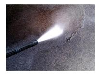
**Clean the surface thoroughly using a jet wash** Then allow to dry. Some damp patches are acceptable but pooling water must not be present.
